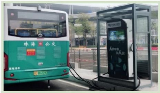
Hong Kong-Zhuhai-Macao Bridge Bus Charging Station
